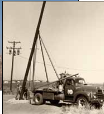
Setting a pole. Both black and white photos to the right are from South Plains Electric.
