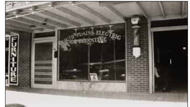
South Plains Electric Cooperative moved to this office space at 1107 Ave. G in Lubbock around 1940.
