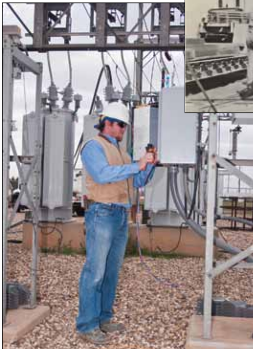
System improvements are a never-ending task for the Cooperative. Eric Garza, left, works on upgrades at the Frenship substation.
