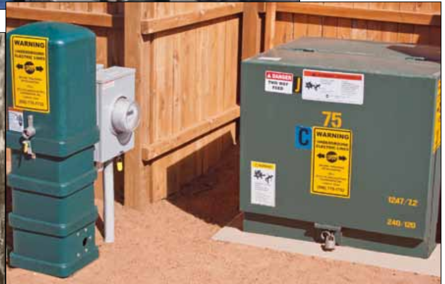
Today, modern residential meters are located in the alleys and are read remotely from the office, saving time and money. The two-way communication is via our power lines, and is safe and reliable.
