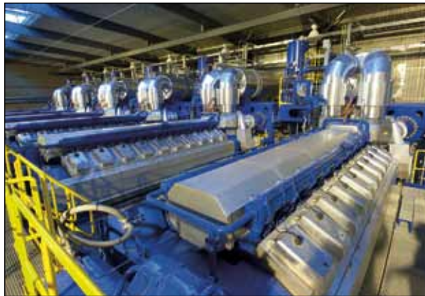
Antelope Station, located in Abernathy, Texas, is a source of quick-start, natural gas-fired generation with 18 Wartsila reciprocating engine generators. Because the Wartsila engines start quickly, are fuel efficient and use little water, they are the perfect supplement to the intermittent wind produced from the Wind Ranch.
