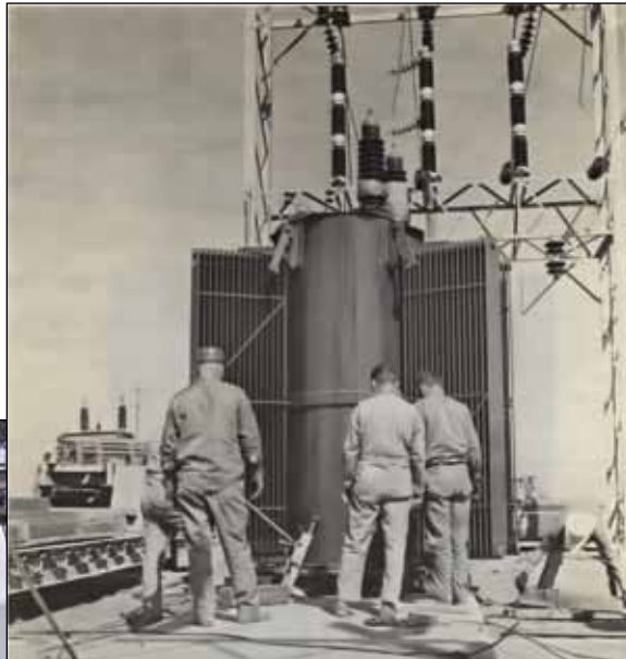
The Cooperative installed a 7,500 KVA transformer at the Woodrow substation in 1966. The transformer had more power capacity than did the entire system in 1938.
