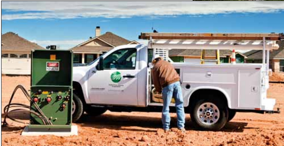
Robert Lueb prepares the new underground service on a Betenbough subdivision in Southwest Lubbock, pictured above.
