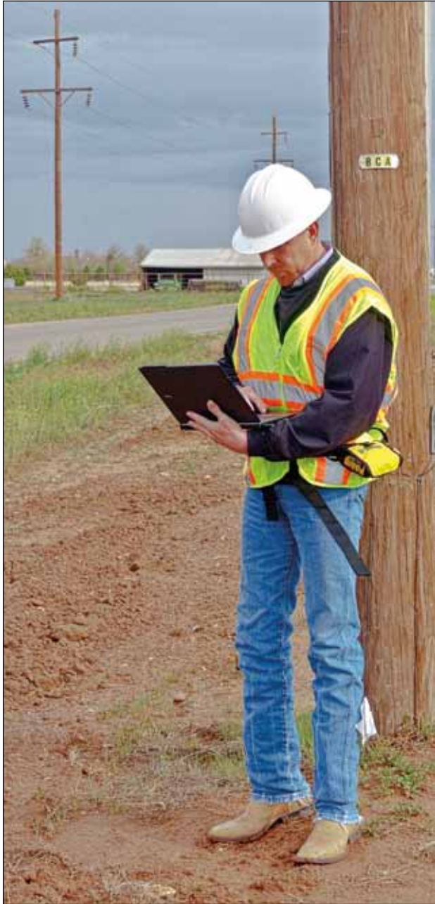
Brad Swaffar uses a computer to wirelessly stake a new electric service using global positioning technologies.
